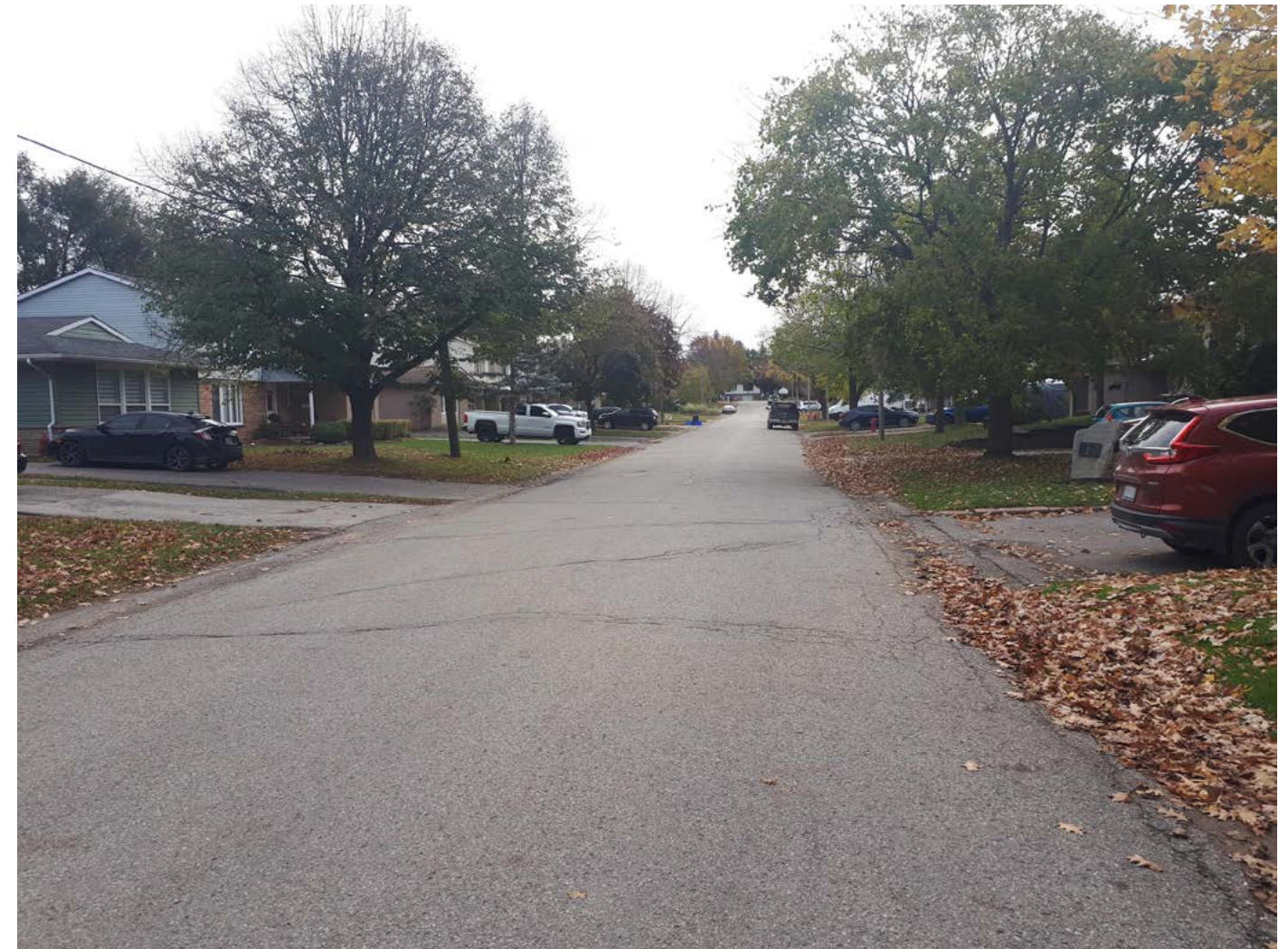
Y:\Public Works Department\Budget\2019\Budget Pictures\Final Pics\B0085.0000 b Cardwell St Reconstruction Princess to Dufferin.jpg
