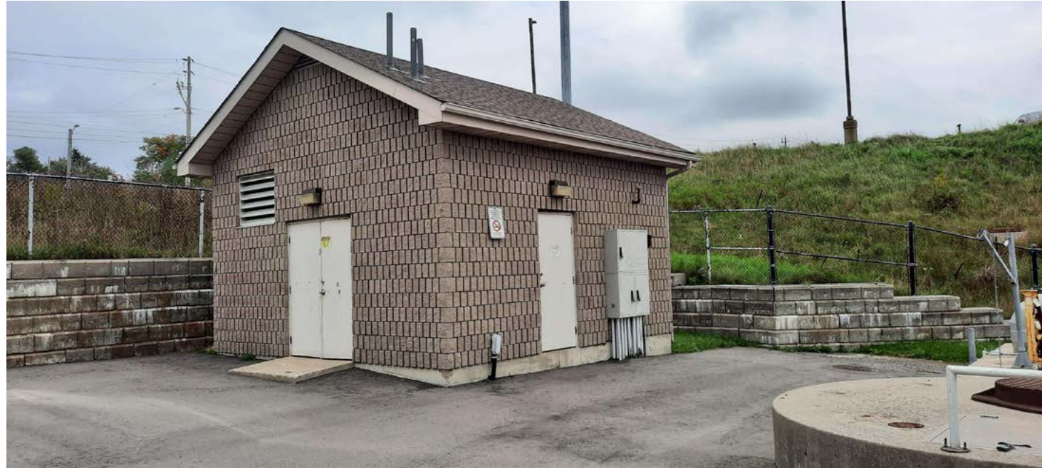
Buena Vista Sewage Pump Station
