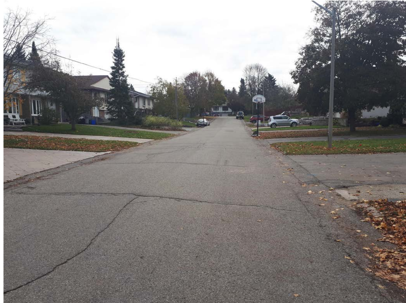
Y:\Public Works Department\Budget\2019\Budget Pictures\Final Pics\B0085.0000 a Cardwell St Reconstruction Princess to Dufferin.jpg
