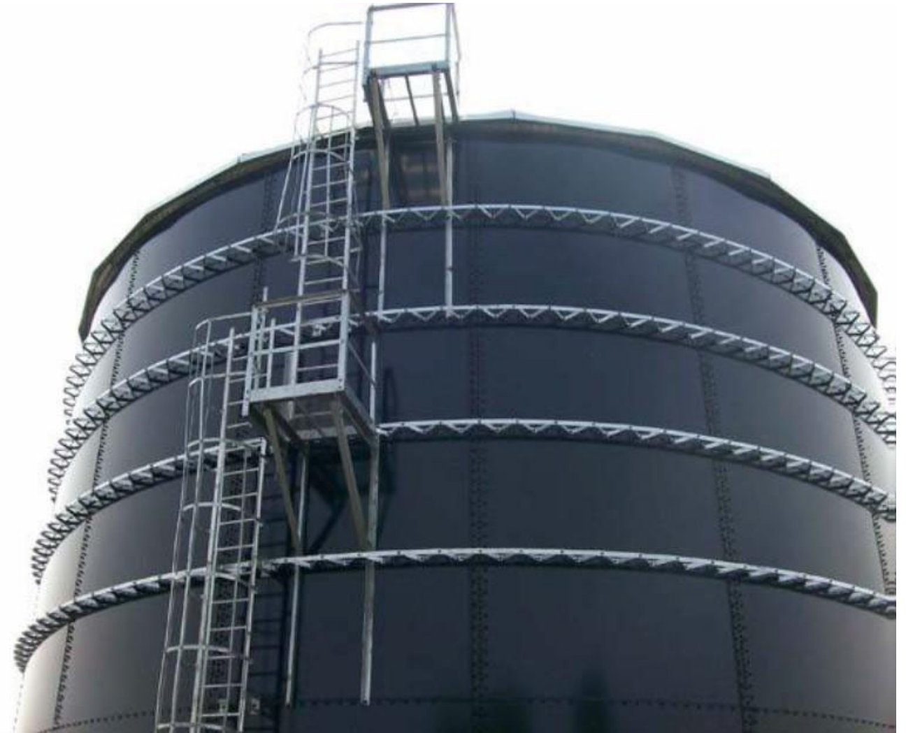
Water Storage Facility - Well 5/5A site
