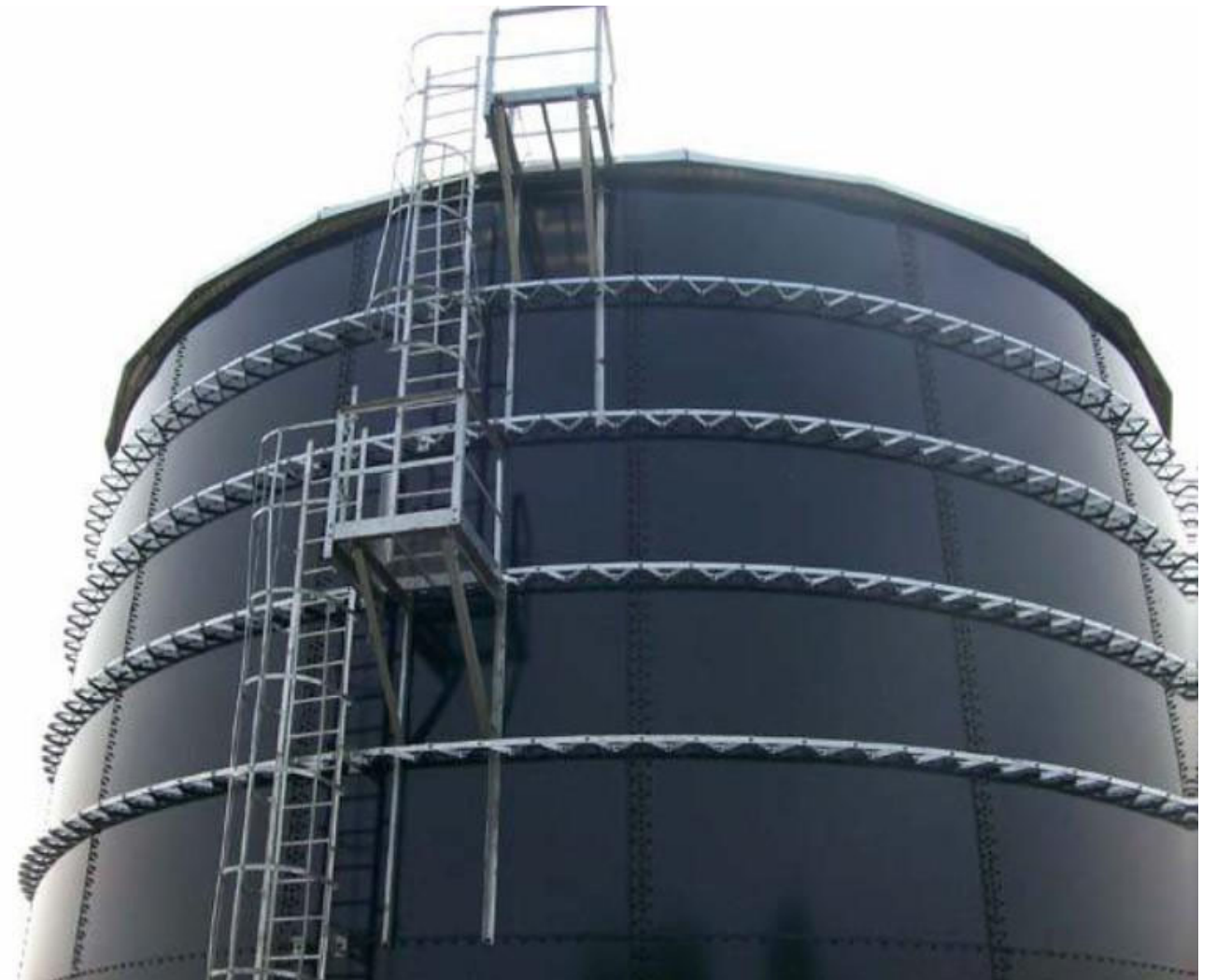
Water Storage Facility - Well 5/5A site
