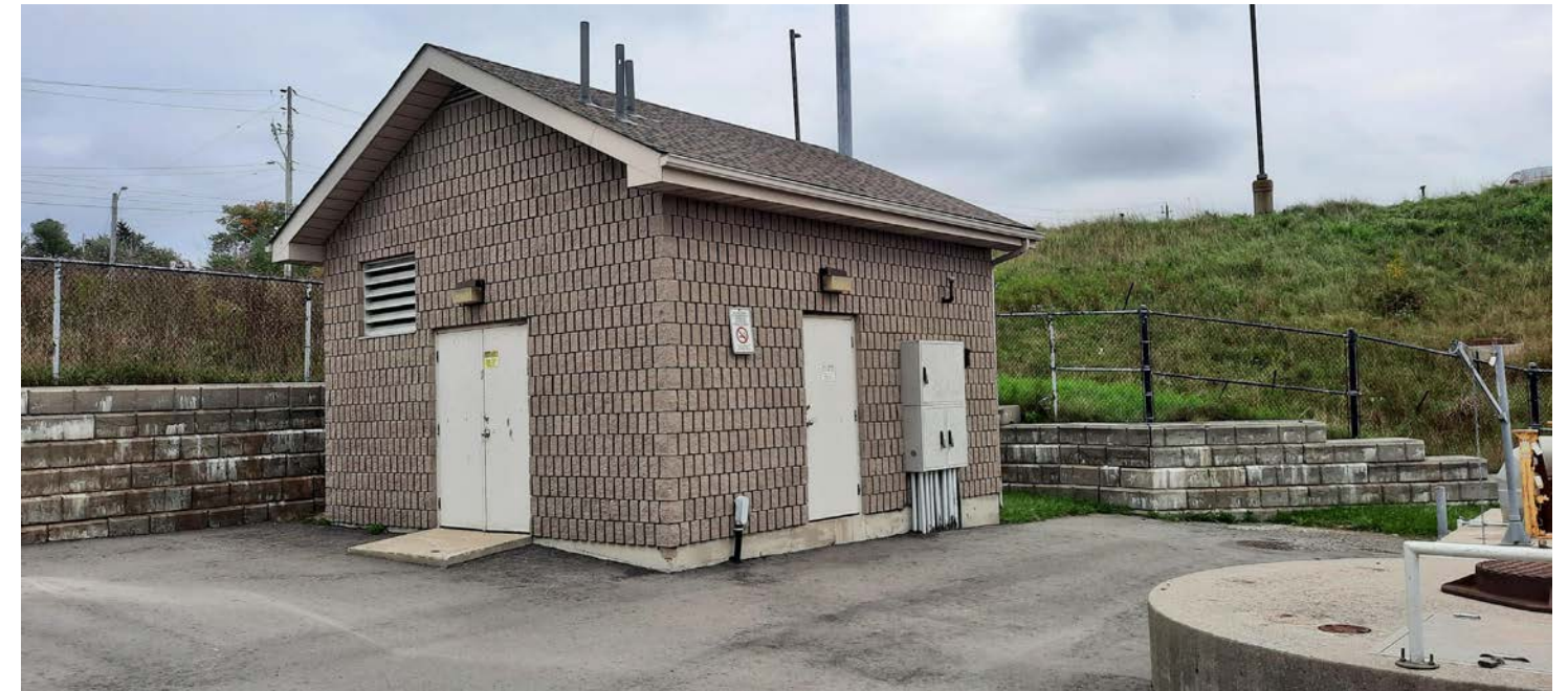
Buena Vista Sewage Pump Station
