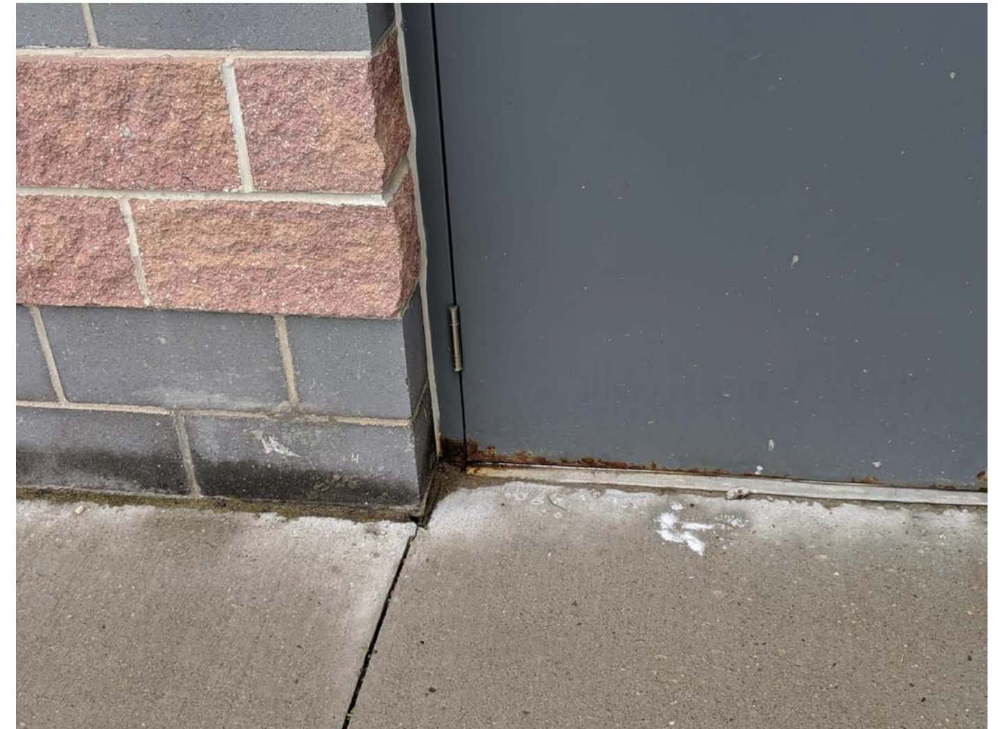
C:\Users\ccosgrove\Town of Orangeville\Facilities - Recreation Facilities\Capital Budget Pictures 2020\Alder Exterior Doors.jpg
