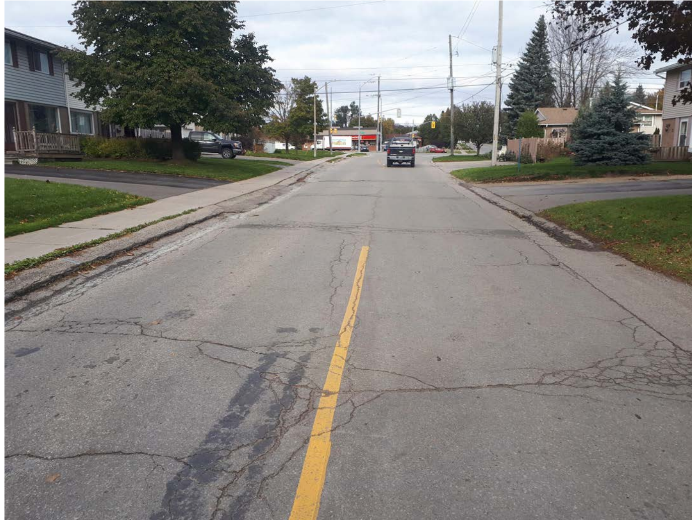
Y:\Public Works Department\Budget\2019\Budget Pictures\Final Pics\B0084.0000 Cardwell Street Reconstruction Princess Street to Townline.jpg
