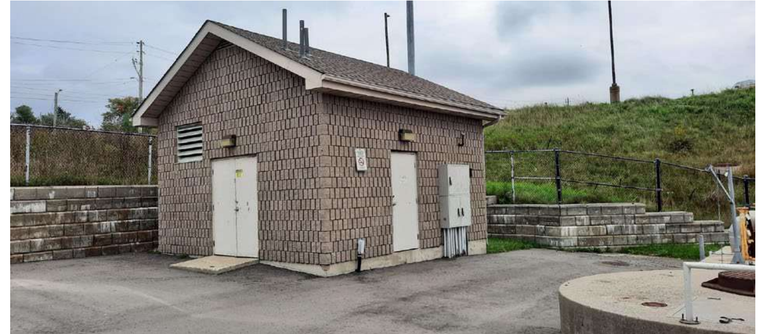
Buena Vista Sewage Pump Station
