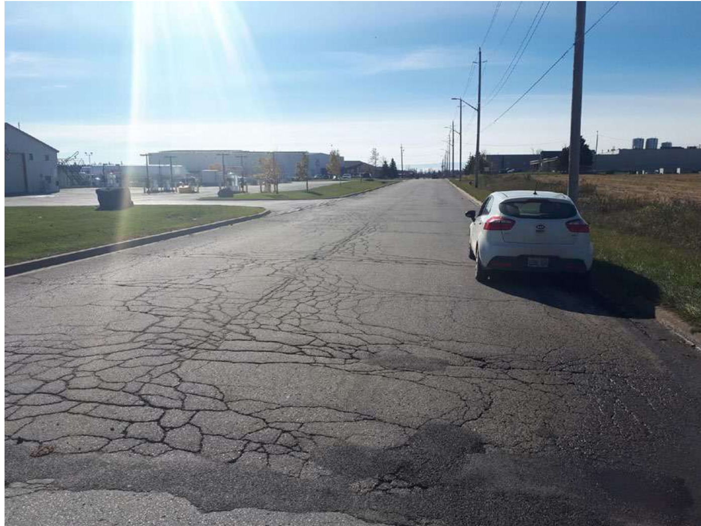
Y:\Public Works Department\Budget\2019\Budget Pictures\Final Pics\B0797.0000 a Richardson Road Rehabilitation.jpg
