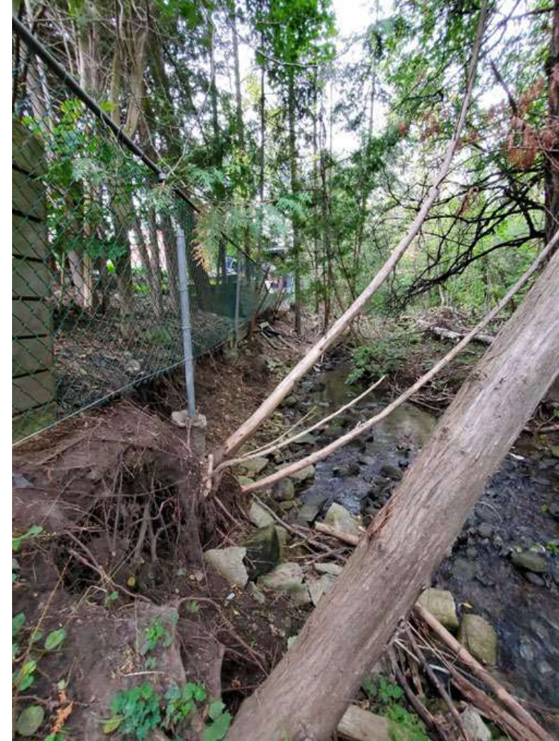
C:\Users\lccosgrove\Documents\2022 Budget pictures\Monora Creek washout 215 Kensington Place\Monora Creek 5.jpg
