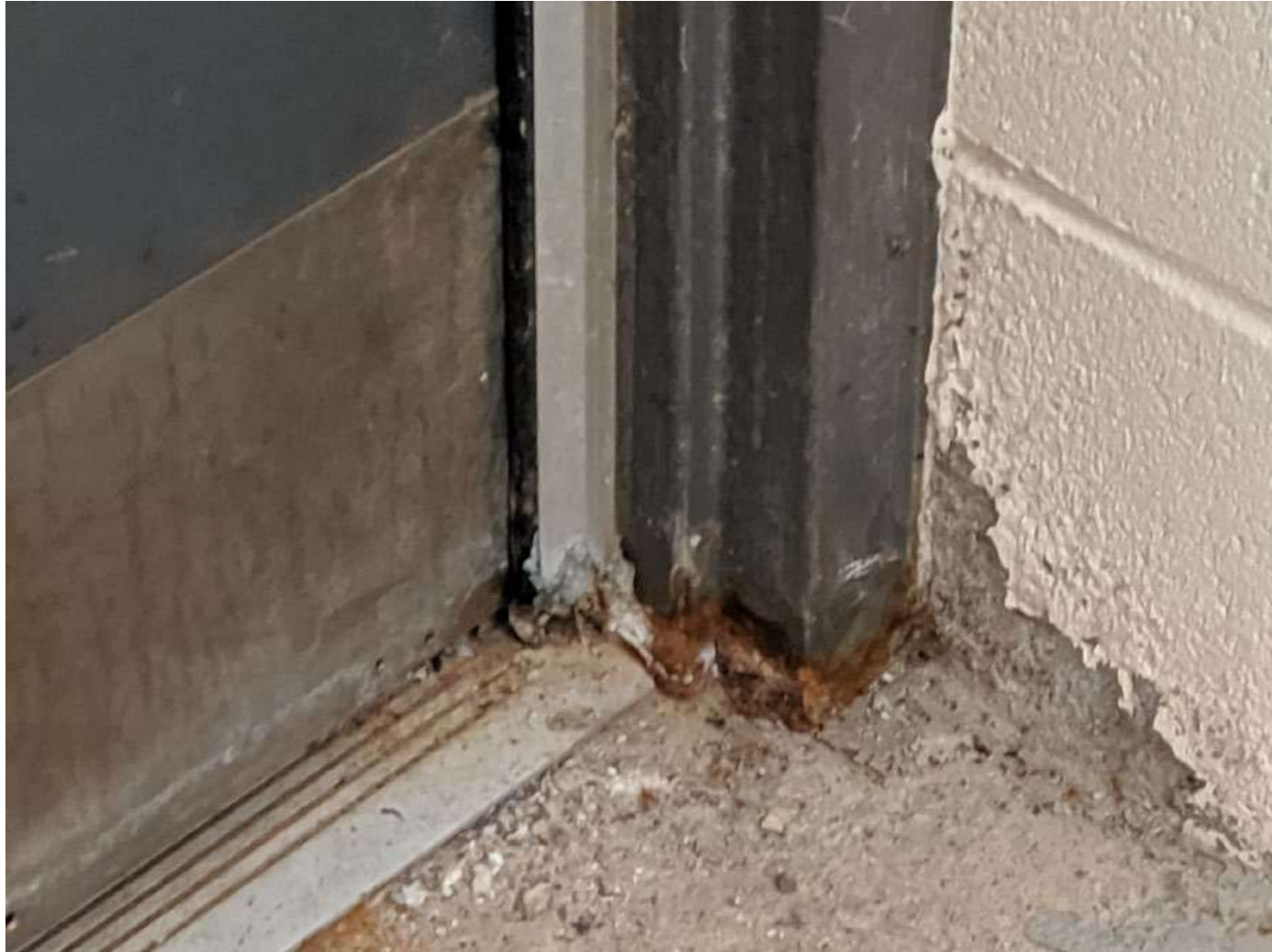
C:\Users\ccosgrove\Town of Orangeville\Facilities - Recreation Facilities\Capital Budget Pictures 2020\Alder Exterior Door 4.jpg
