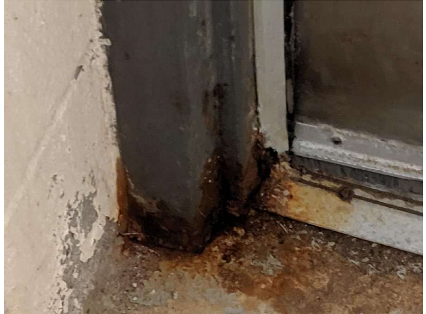
C:\Users\ccosgrove\Town of Orangeville\Facilities - Recreation Facilities\Capital Budget Pictures 2020\Alder Exterior Door 5.jpg
