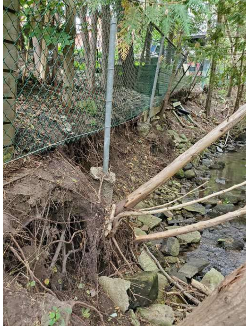
C:\Users\lccosgrove\Documents\2022 Budget pictures\Monora Creek washout 215 Kensington Place\Monora Creek 4.jpg
