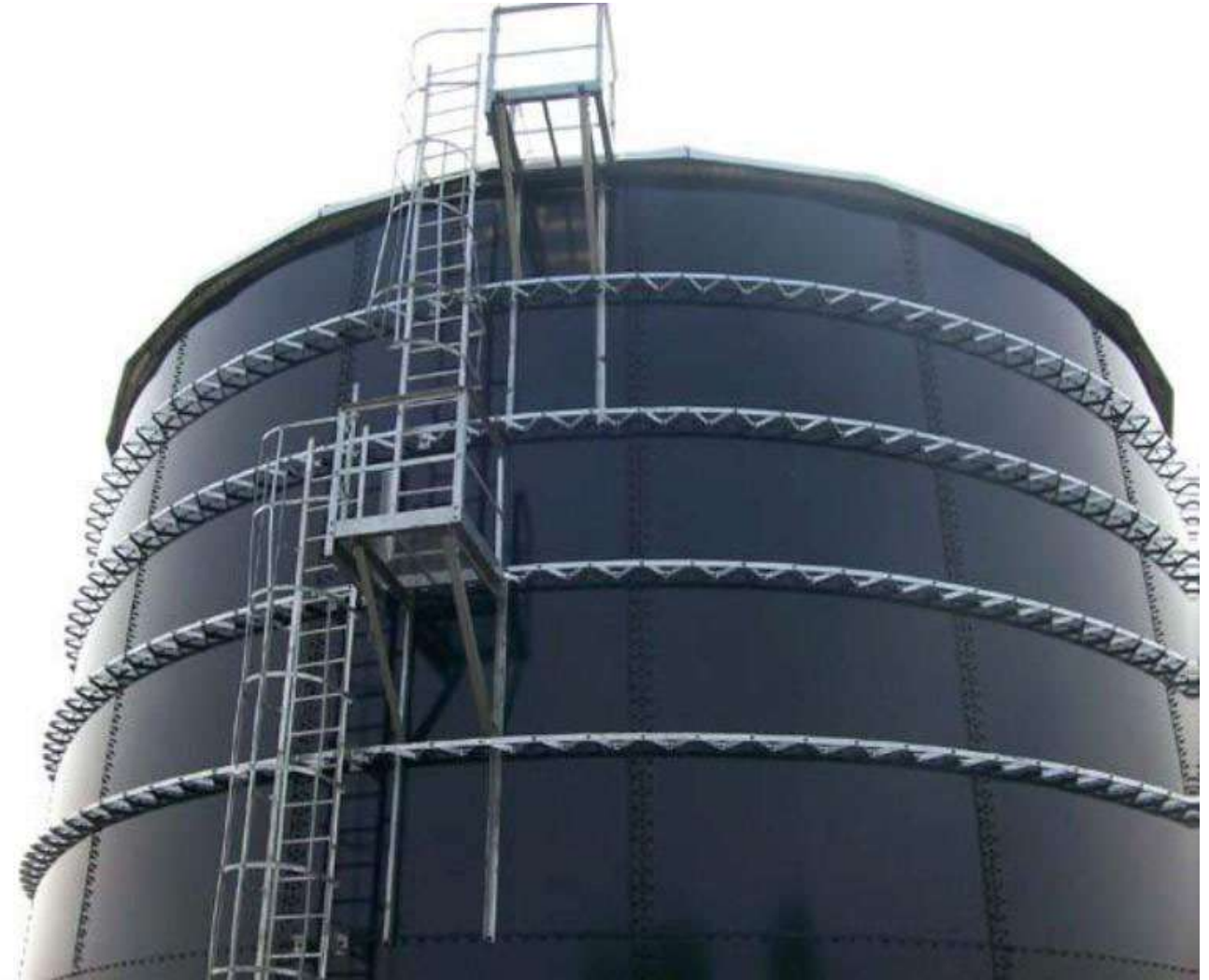
Water Storage Facility - Well 5/5A site
