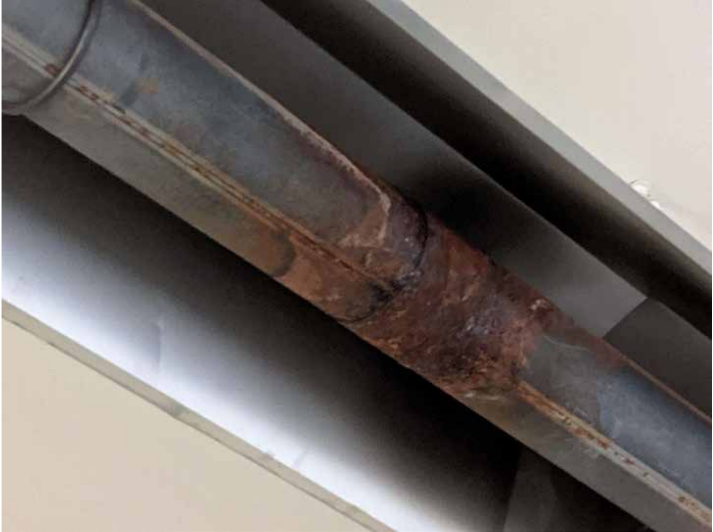
C:\Users\ccosgrove\Town of Orangeville\Facilities - Recreation Facilities\Capital Budget Pictures 2020\Alder Green Rink Heater.jpg
