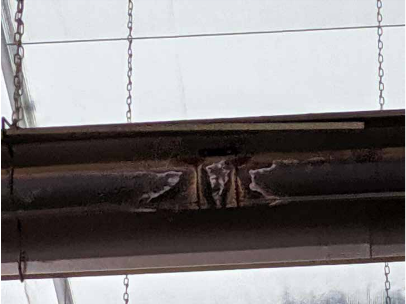
C:\Users\ccosgrove\Town of Orangeville\Facilities - Recreation Facilities\Capital Budget Pictures 2020\Alder Red Rink Heater three.jpg
