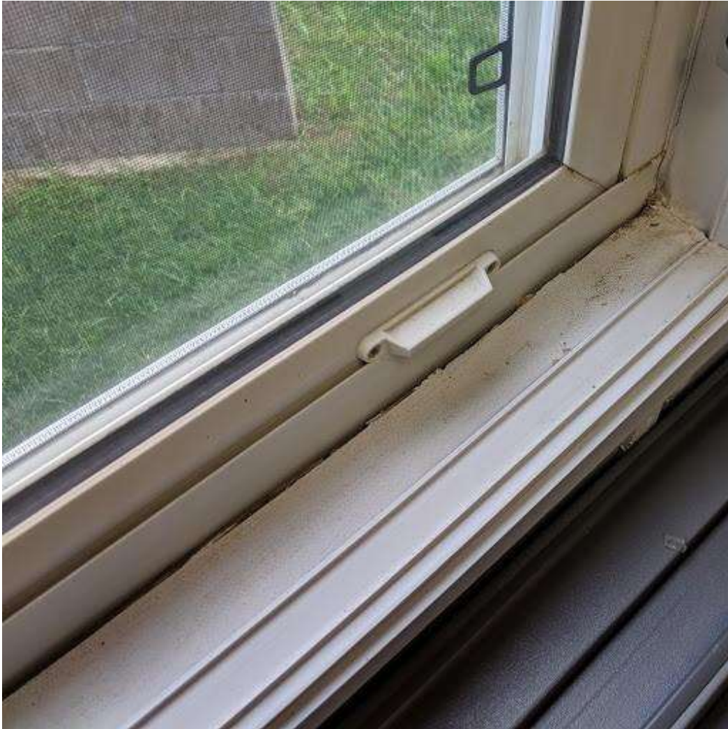
C:\Users\ccosgrove\Town of Orangeville\Facilities - Corporate Facilities\Capital Budget Pictures 2020\Diane Drive Windows 3.jpg
