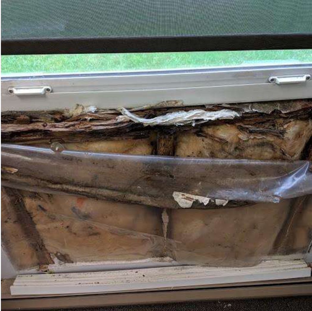
C:\Users\ccosgrove\Town of Orangeville\Facilities - Corporate Facilities\Capital Budget Pictures 2020\Diane Drive Windows 4.jpg
