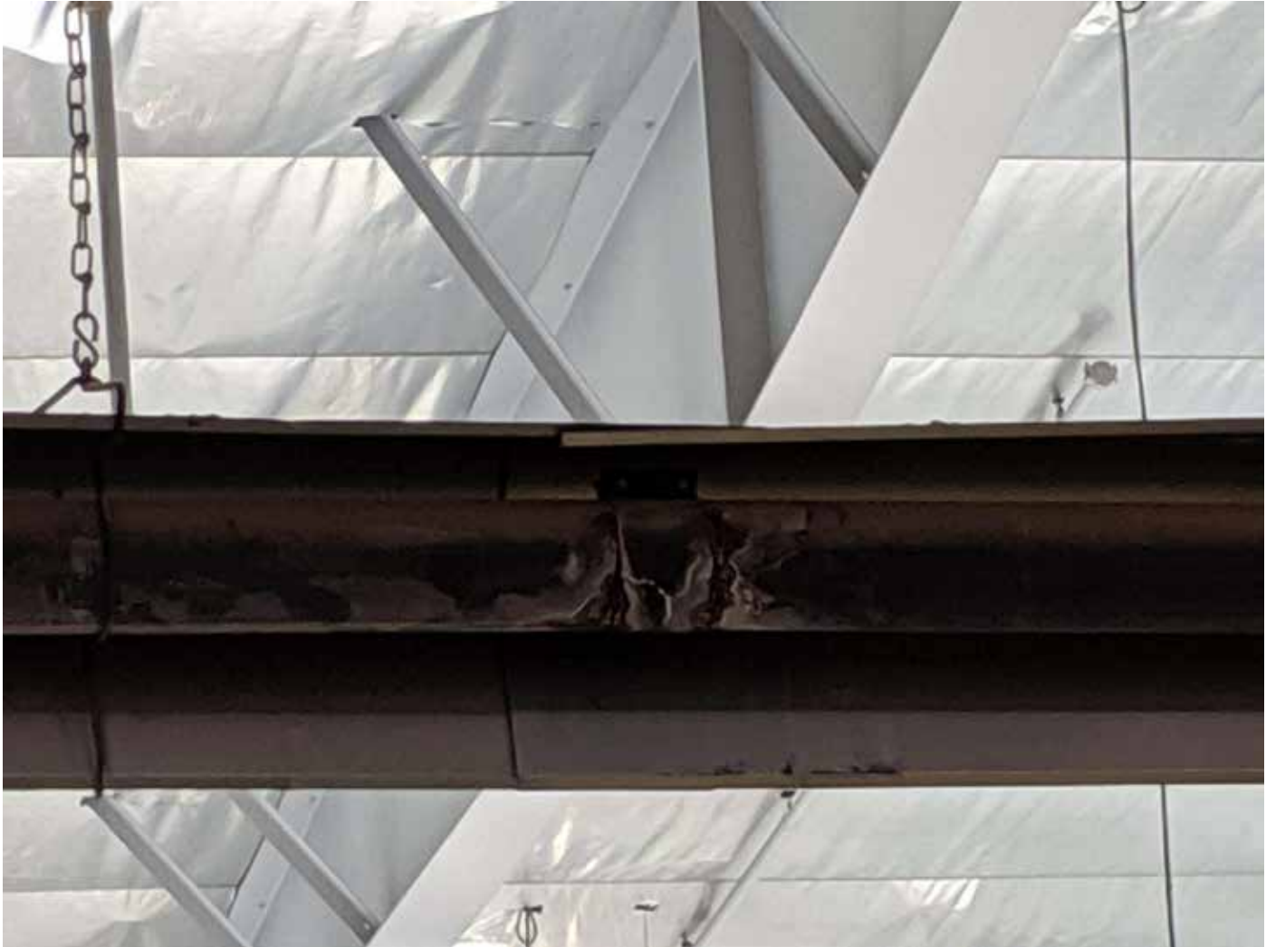
C:\Users\ccosgrove\Town of Orangeville\Facilities - Recreation Facilities\Capital Budget Pictures 2020\Alder Red Rink Heater.jpg
