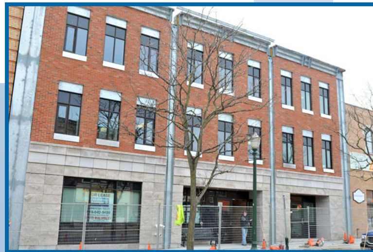
Construction on the new Wellington-Dufferin-Guelph Health Unit commenced in 2013.
