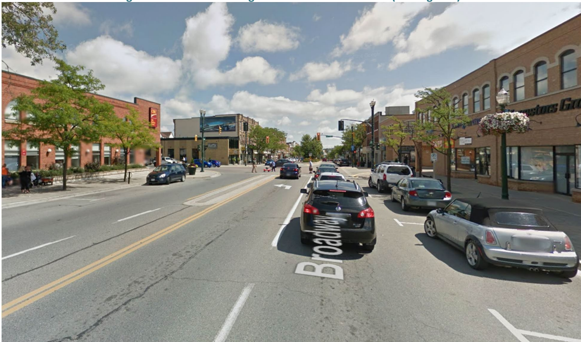
Figure 5: Downtown Orangeville Transit Terminal Site (looking east)
