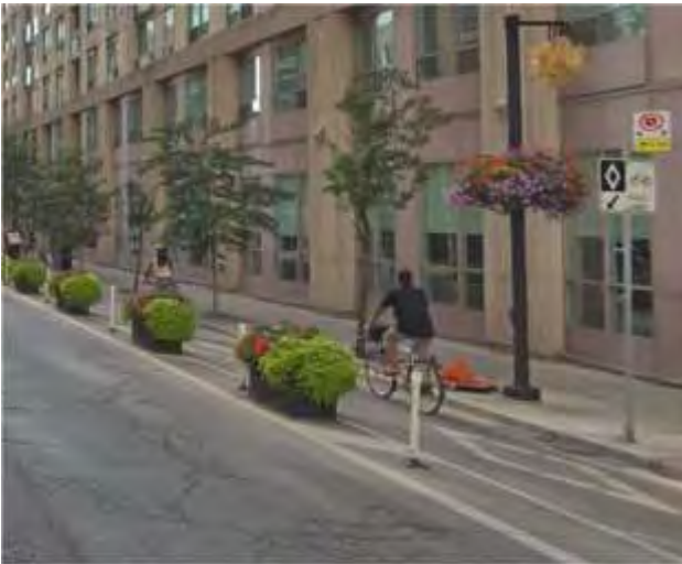
Buffered Bicycle Lane (physical buffer with flexible bollards, planter boxes)
