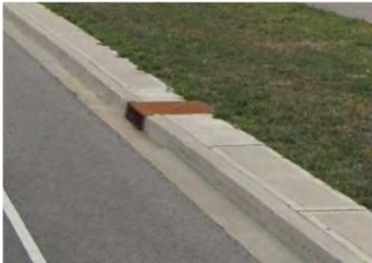
Example of Curb Inlet Catch Basin
