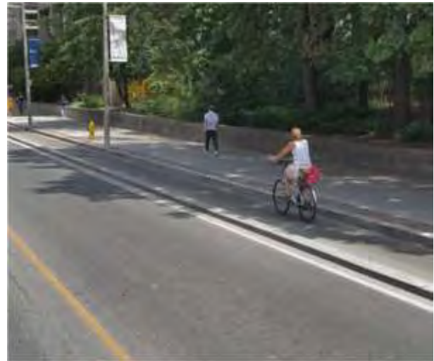
Buffered Bicycle Lane (physical buffer with a concrete curb)
