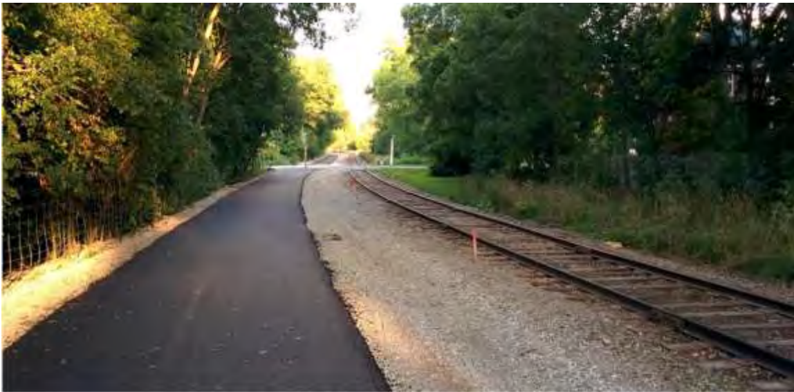
Example of Rail-With-Trail - Waterloo Spur Line Trail
