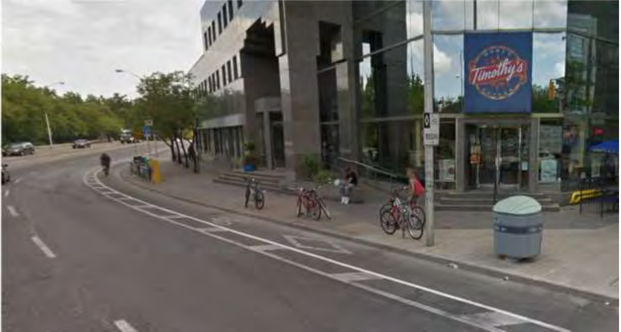
Buffered Bicycle Lane (painted buffer with diagonal hatching)
