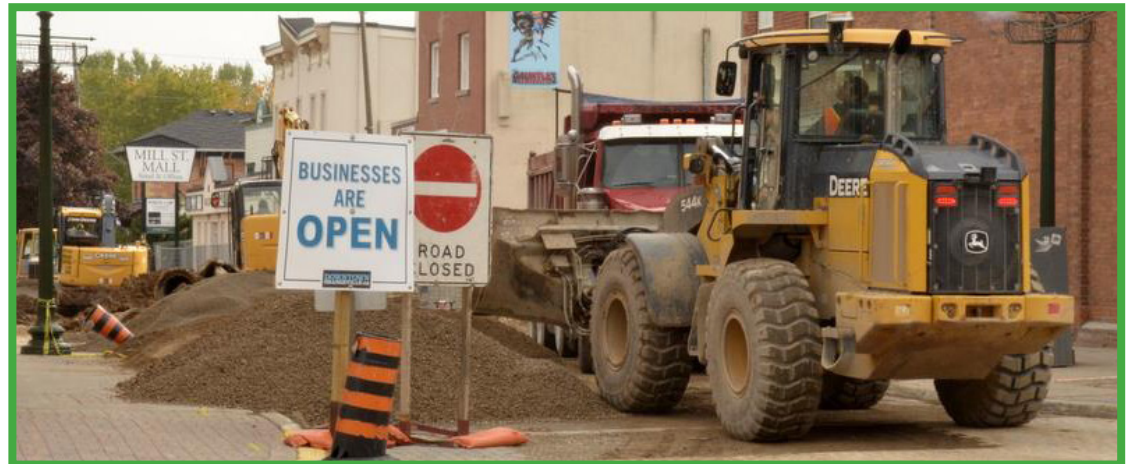
Construction on Mill Street
