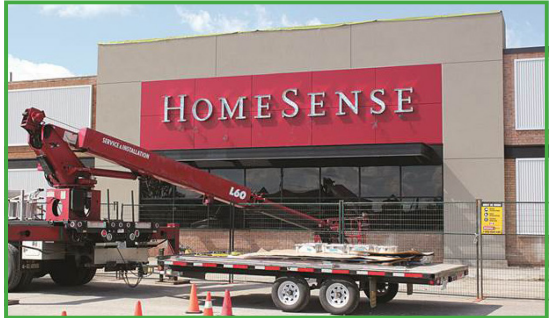
Home Sense underwent renovations
