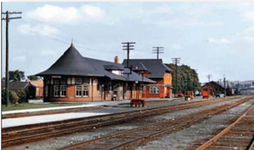
Train Station at Orangeville Rail Yard
