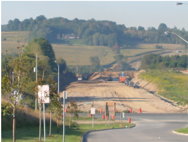
South Arterial Road Construction
