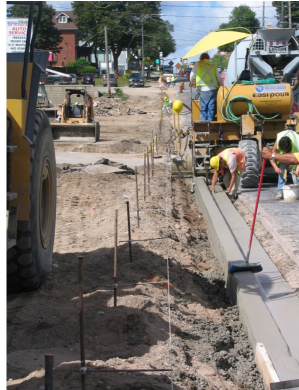
East Broadway Construction
