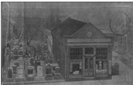
Early Façade Monument Works Building
