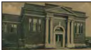
Original Mill Street Façade
