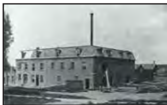
The Casket Factory & Planing Mill
