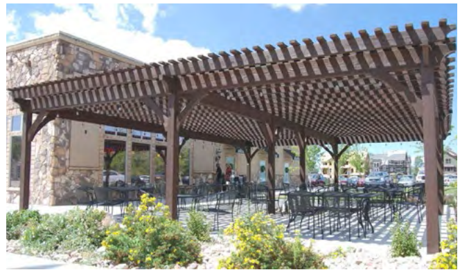
A architecturally designed shelter creates an interesting and comfortable outdoor amenity space.
