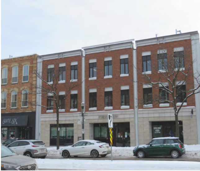
Example of a new build which incorporated architectural detailing that successfully breaks the building mass into three separate components, in keeping with the scale of surrounding development.
