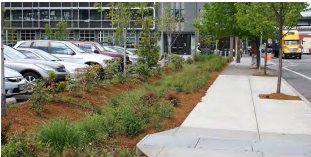
Example of parking boiawale and landscape screening strip to buffer parking area.
