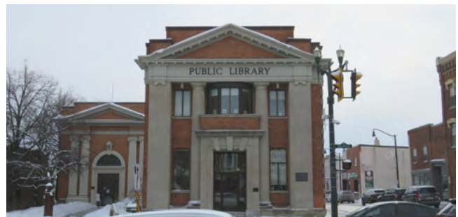
Examples of vertical elements framing the entrance and providing visual interest to the façade.
