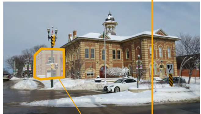
EXAMPLE OF AN ADDITION LOCATED TO THE SIDE/REAR YARD AWAY FROM PRIMARY ELEVATION
