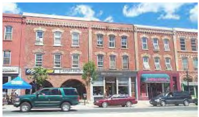
Example of storefront cornice maintaining visual appearance and height.
