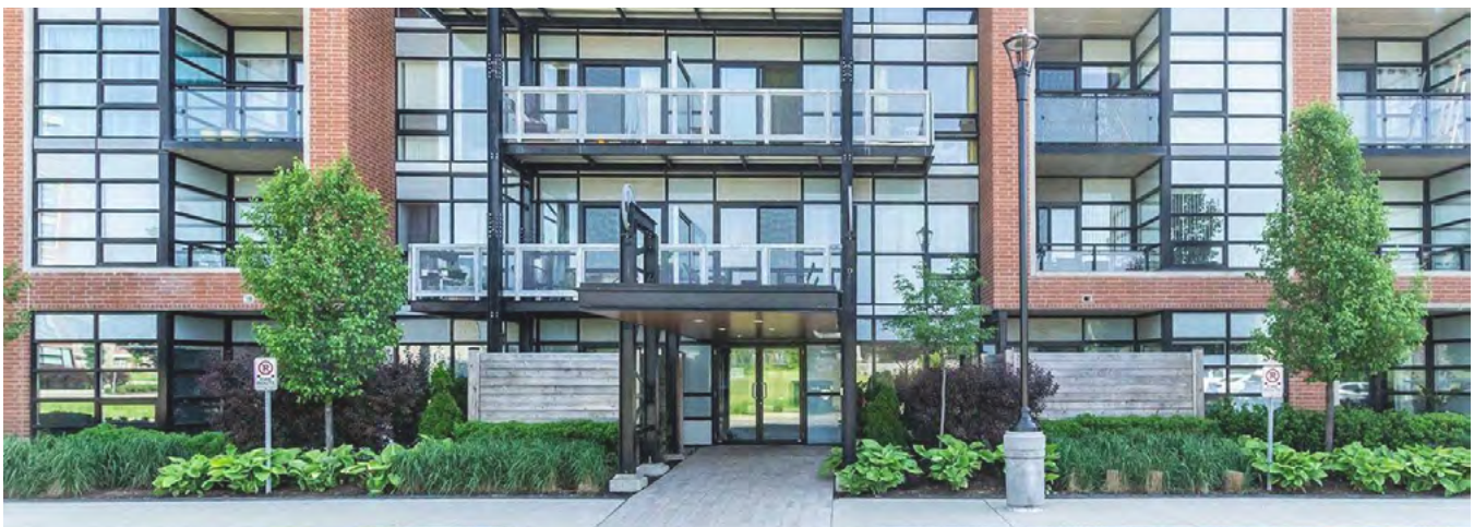
Use of high quality materials including a large amount of glass and a comfortable pedestrian environment.
