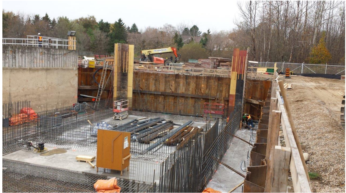
Construction of the New Bioreactor
