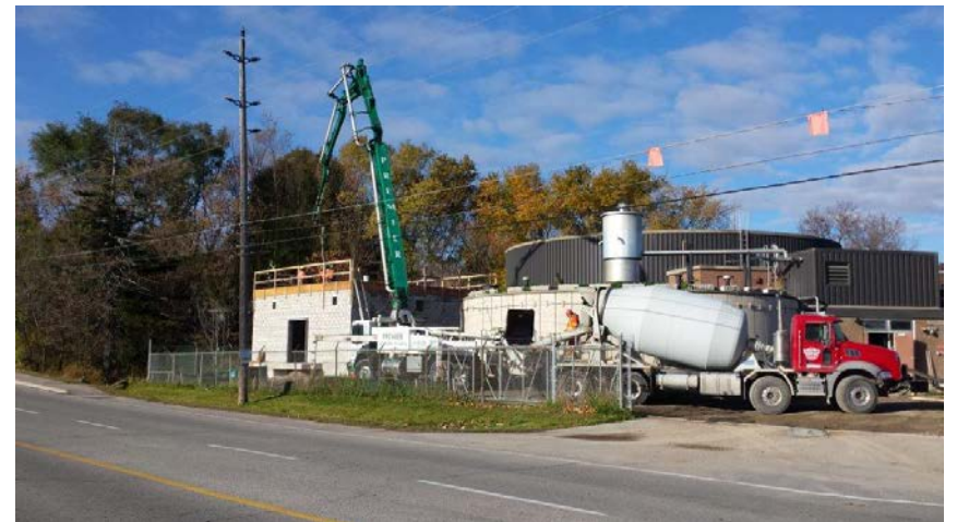
Construction at the Water Pollution Control Plant
